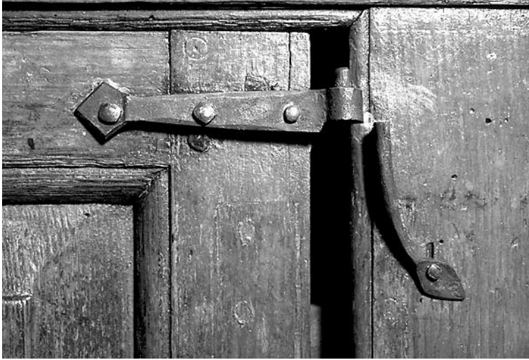
Figure 7. Close-up view of cupboard hinge with the door moved slightly to one side to show the cut hinge pintel.
