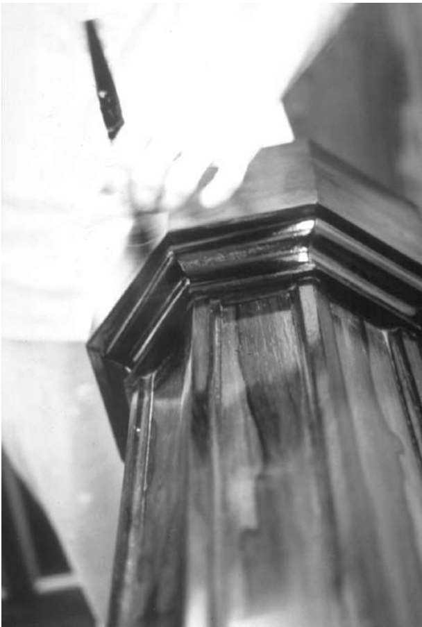
Handbrushing twelve coats ultralight dewaxed shellac.
