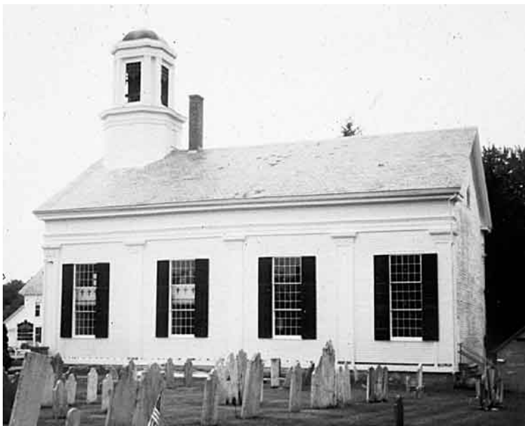
Figure 10. The Cornwall Congregational Church. The passive improvements made in this building had no effect on its appearance.
