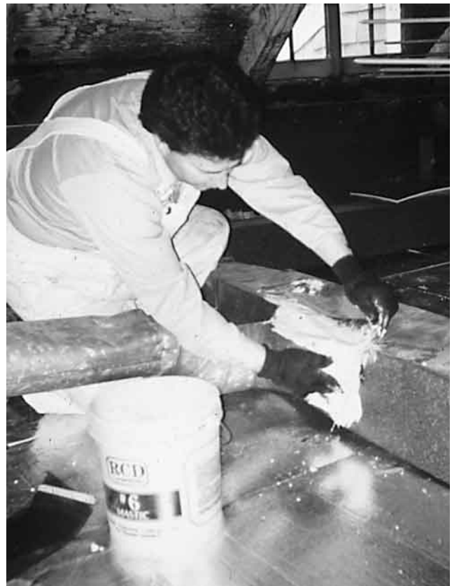
Figure 7: Sealing a duct with duct mastic.
