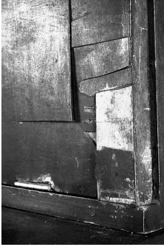
Figure 5. Close-up of a projecting batten and associated veneer damage on the warped fallboard in figure 4, before treatment.
