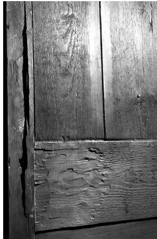
Figure 10. A close-up of damage on the reverse caused by the force of the warping panel (Case Study 4). The stile and rail were initially weakened by early adze cuts which provided chimney clearance for the panelling.
